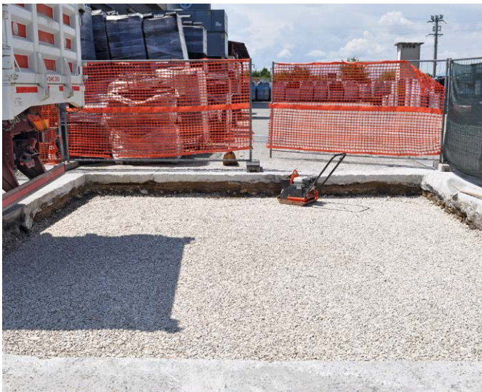
Figure 9: laying aggregate for base layer
