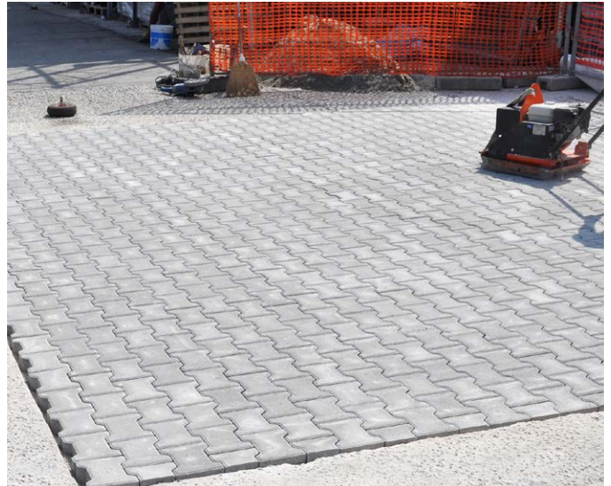
Figure 15: compacting the interlocking pavement blocks
