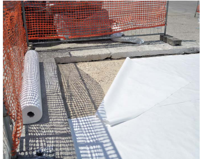
Figure 10: laying the geotextile on the aggregate layer
