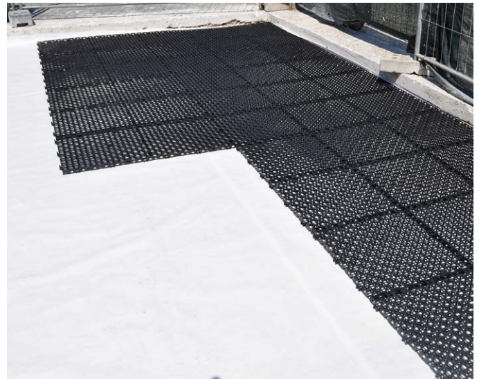
Figure 11: laying the Geocell panel
