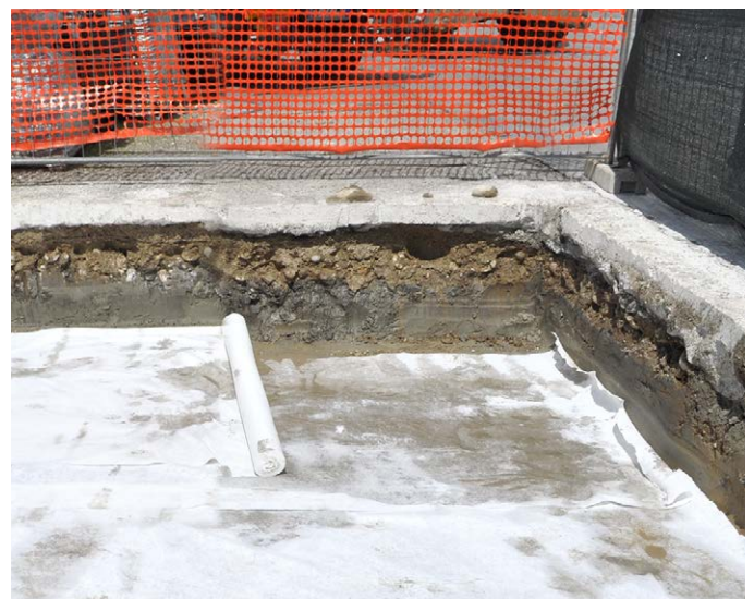
Figure 8: laying the geotextile on the excavation base
