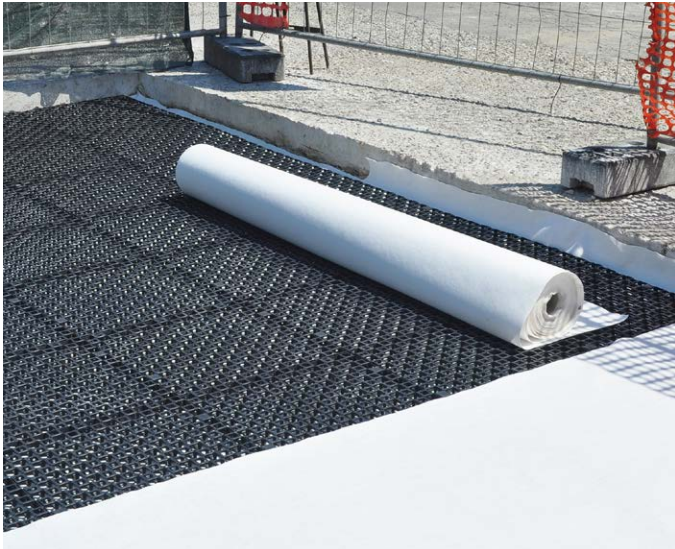
Figure 13: laying the geotextile above the Geocell
