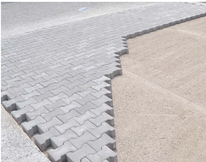
Figure 14: laying the sand setting bed and the interlocking pavement blocks
