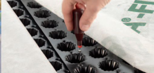
Joining sheets with DELTA®-FLORAXX connecting elements.
